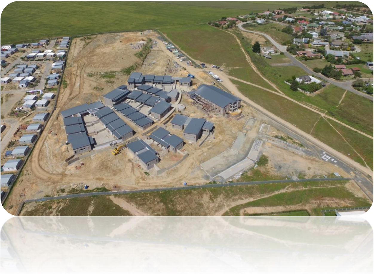
New School in Tulbagh
